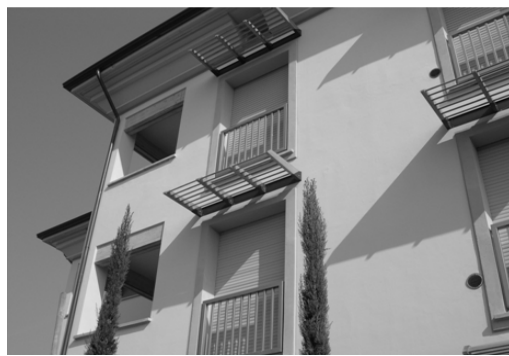
The Ozzano project – Bologna (IT) Social Housing organization: COPALC 12 eco-dwellings Construction: May 2005 / December 2006
