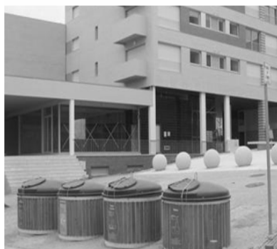
The Matosinhos project – Porto (PT) Social Housing organization: NORBICETA 101 eco-dwellings Construction: December 2004 / February 2007
