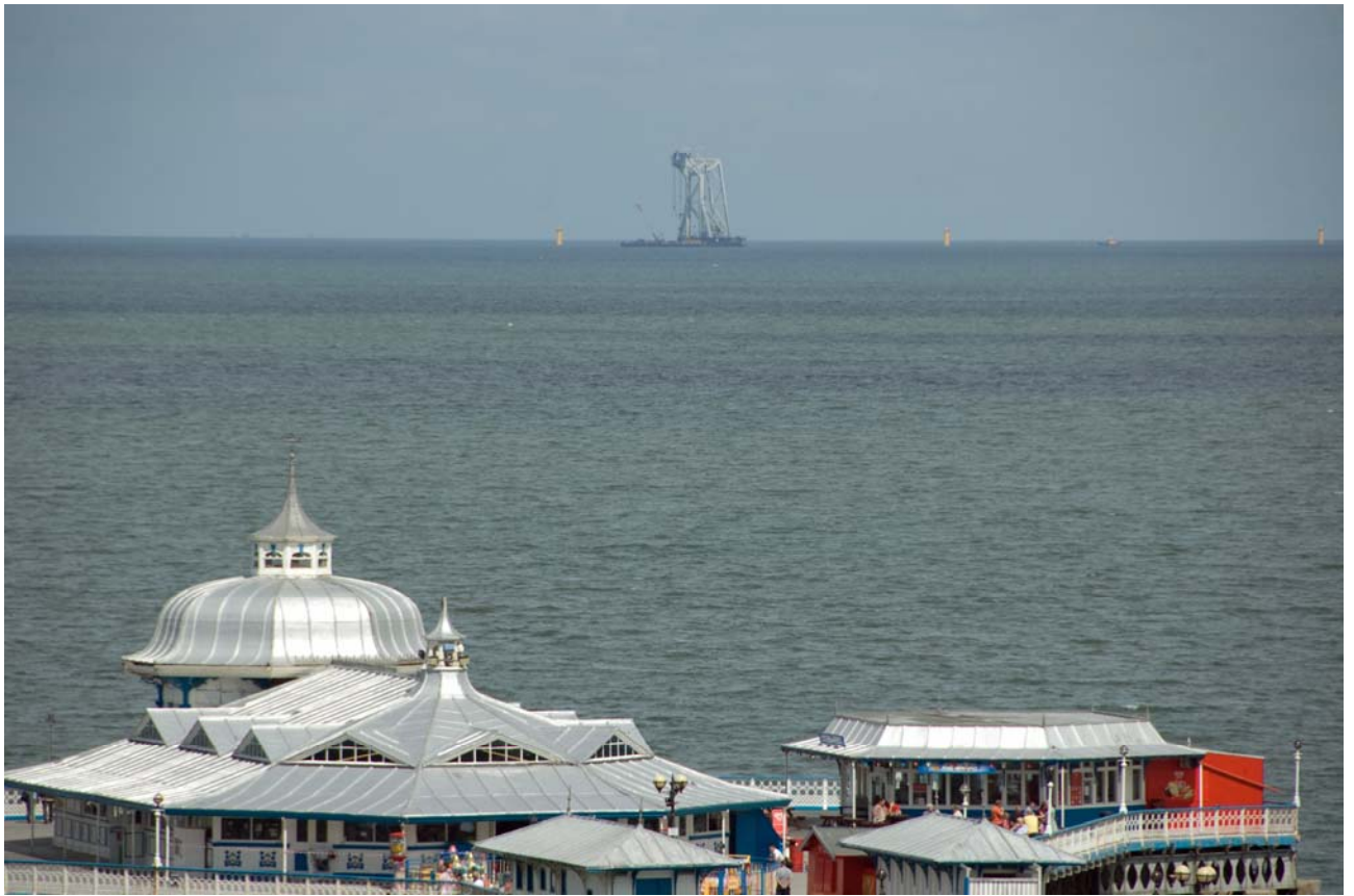
HLV SVANEN off Llandudno Pier – installing Turbine Bases
