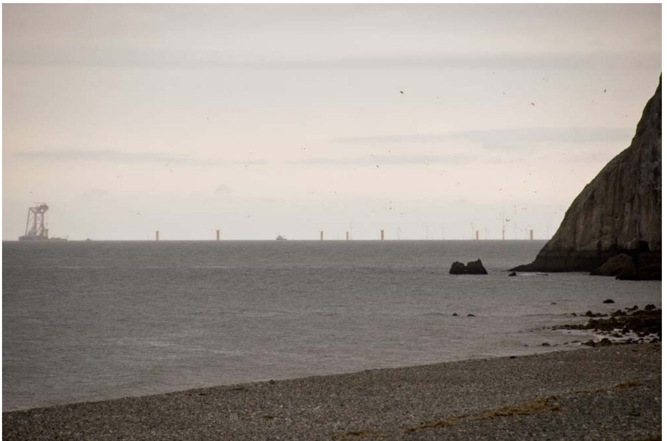
HLV SVANEN off the Little Orme – installing Turbine Bases
