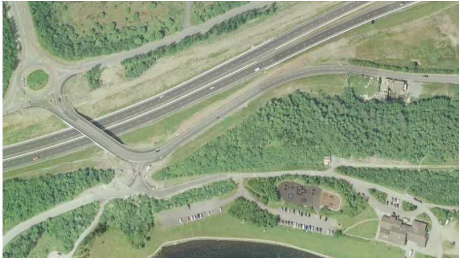
Figure 2. Merthyr Road on approach to Tafarnaubach Bridge
